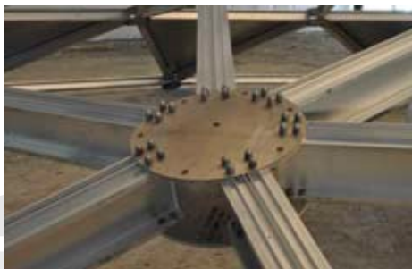
Node detail utilizes proprietary extrusion design.
